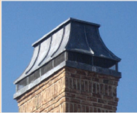
“Wagon” chimney cap shown in 16 oz lead coated copper (Long Island, NY)
