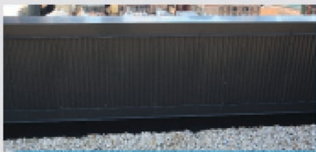
Inner Parapet Wall
